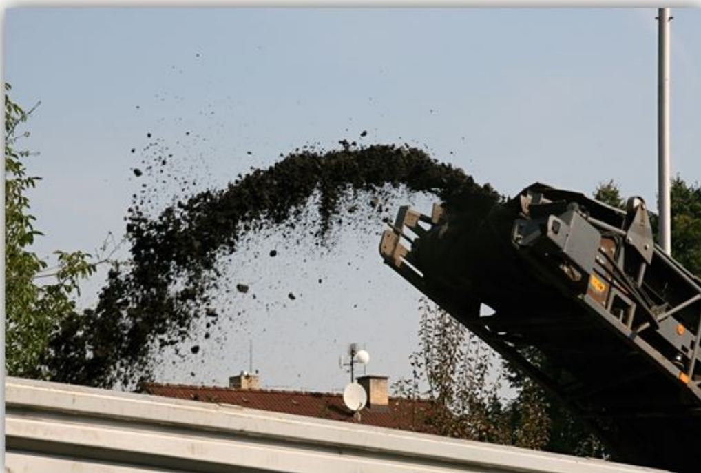
11 TAKHLE SE TO SYPE
